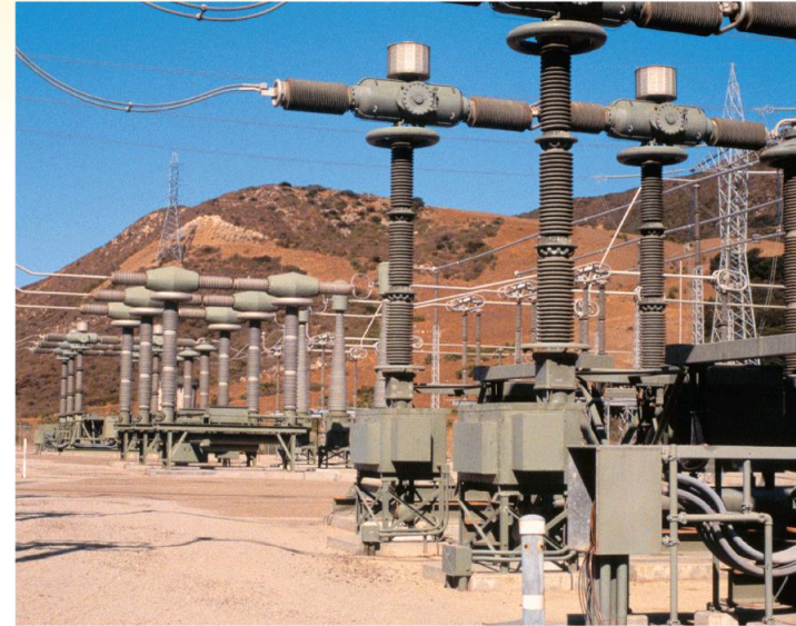
B Step-up Transformer
